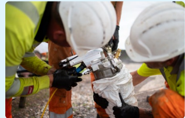
Operators inflating the sewer liner
